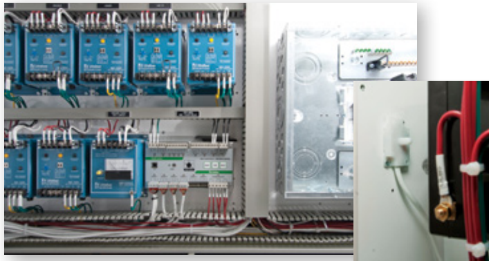
Figure 2. Typical installation of the PGR-8800 Arc-Flash Relay and the light sensor.
