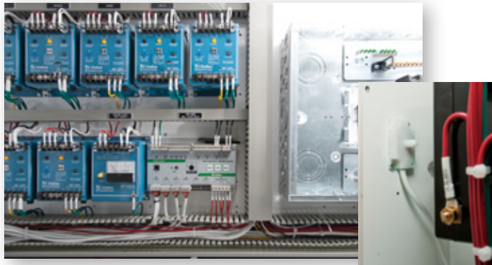
Figure 2. Typical installation of the PGR-8800 Arc-Flash Relay and the light sensor.
