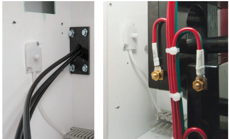
Examples of appropriate point sensor installation.
